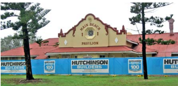
Hutchies at work on the landmark pavilion.
